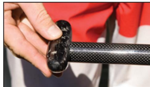
3) Insert the handle onto the shaft. Line up the flat side of handle with the outward facing blade while the epoxy is still wet.
